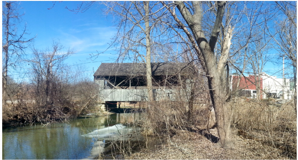
BUFFALO CREEK • SPRING The Long Grove covered bridge from the creek bank — cedar siding from the 1970's wrapped around iron from 1902. The cover is a faithful copy of the famous covered bridge in Ashuelot, New Hampshire.
