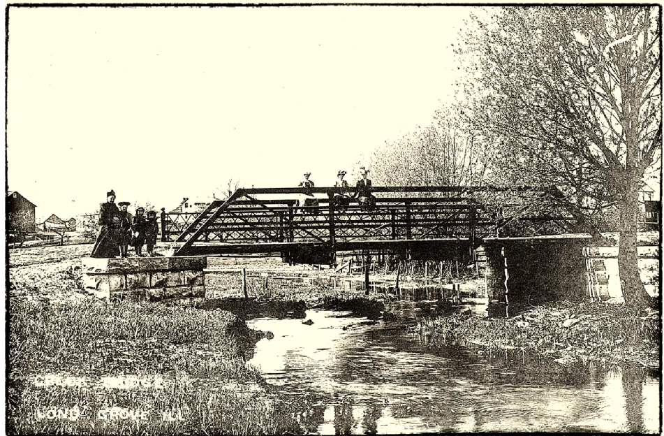
BUFFALO CREEK · 1908 The Long Grove iron-truss bridge in 1908, taken from a photo postcard. The back of the postcard reads — "Just enjoying a long sweet smoke at the corners."
