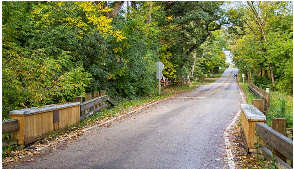
PLATE I The Founders Memorial Bridge on Cuba Road, dedicated to Dorothea Huszagh and those who joined in founding the Village of Kildeer and establishing its rural character.
